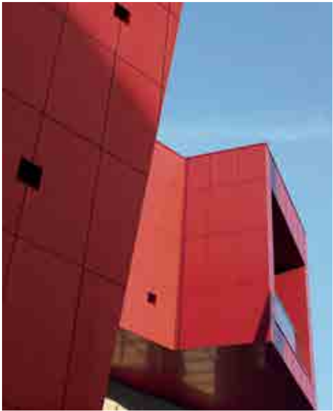
Villa Nesi, Progetto Archibsang Lab + Ing. Alberto Perino, Facciata Ventilata Marazzi Engineering Villa Nesi, Archibsang Lab + Ing. Alberto Perino Project, Ventilated Wall Marazzi Engineering
